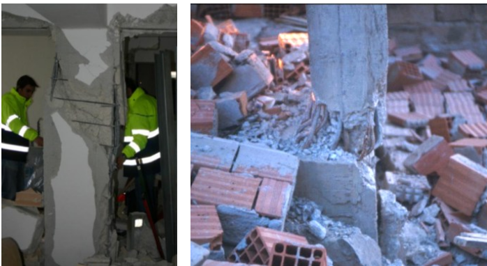
Inadequate capacity and failure (M,V)
