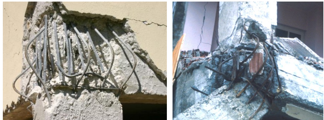
Inadequate shear capacity of the joints
