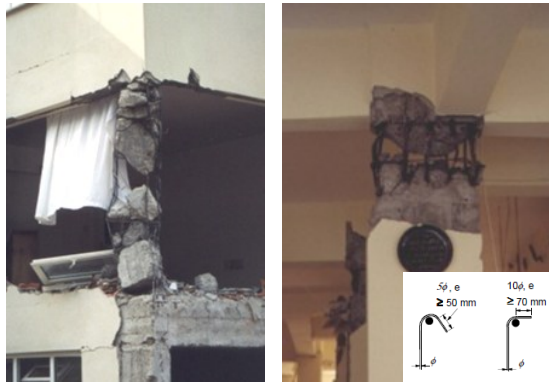
Inadequate capacity and failure (M,V)
